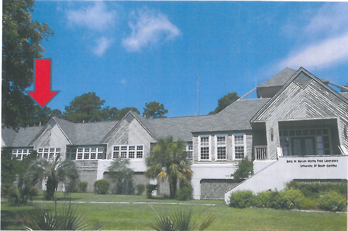
FRONT VIEW OF MARINE RESEARCH FACILITY. RED ARROW SHOWS HVAC LOCATION
